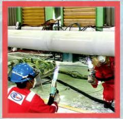
The system uses existing equipment for the abrasive blasting/surface preparation and application of fusion bonded epoxy (FBE) plus chemical modified polypropylene or polyetylene (CMPP or CMPE) dual-powder base layers. The overall thickness required is then achieved by applying powder with a flame spray gun.
